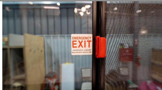
Figure 32. Pull style latch on an emergency exit.
