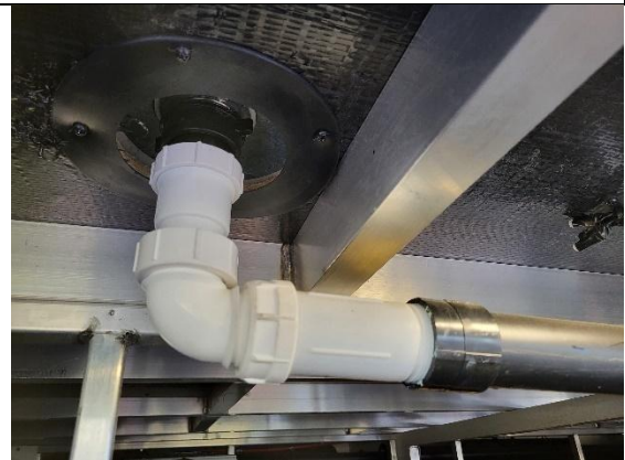
Figure 143. Waterless p-trap under a shower location.
