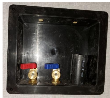
Figure 150. Washer connections and drain.
