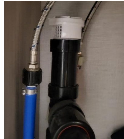
Figure 144. Air admittance valve.
