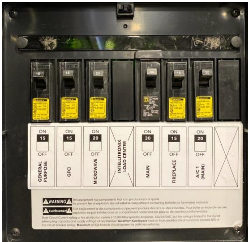
Figure 85. Intellitronix Power Module with 5 circuits installed. The breaker without the yellow label is the input (main) breaker, which would disable all other circuits if turned off.
