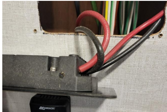
Figure 100. Go Power! Solar Charge controller wiring interface (looking from the top of the controller.). The controller has been removed from the wall and rolled forward.
